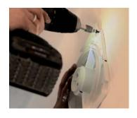
Fix the fan to the wall and make the proper electrical connection
